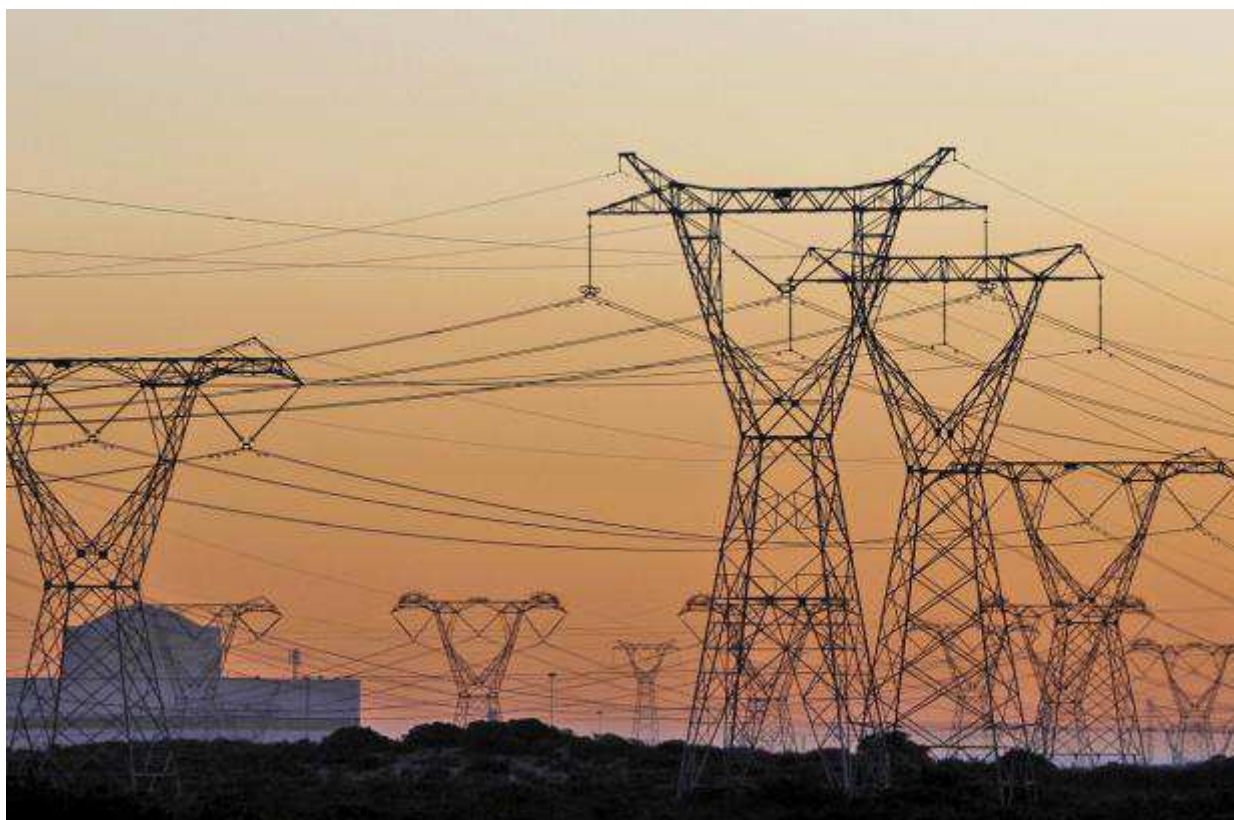
Figure 7: An example of the type of tower structure (namely the 515 series) proposed to support the 400kV power line (internet source: http://www.greenbusinessguide.co.za/eskom-power-supply-tight )
